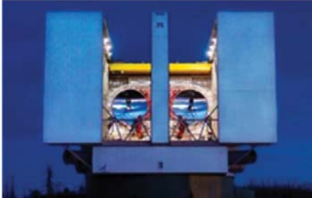
Figure 3. The Large Binocular Telescope 3 on Mt. Graham, Arizona combines two 8.4-m diameter telescopes to achieve excellent resolution and sensitivity, enabling the acquisition of images of planets around other stars. 4
