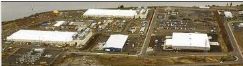
Figure 1. A Google data center; such data centers can hold up to 1,000,000 high performance servers.
