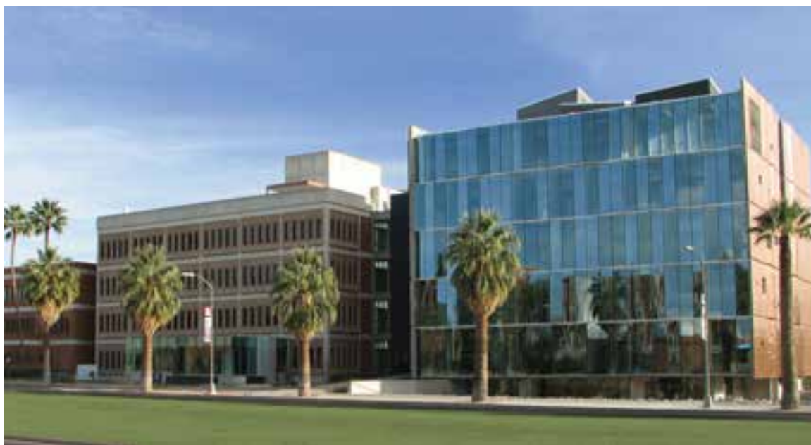
College of Optical Sciences Meinel Building complex, 2010.
