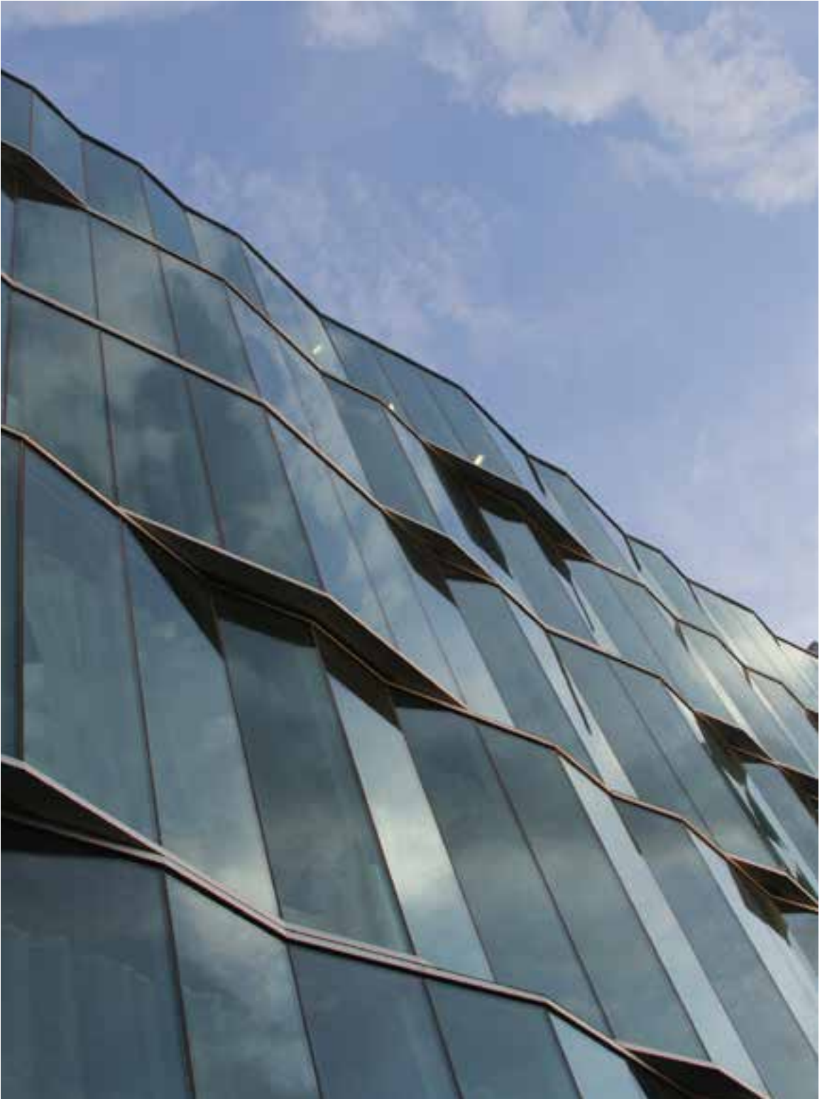
North face of Meinel Building, with clouds. (Photo by R. Dawson Baker)
