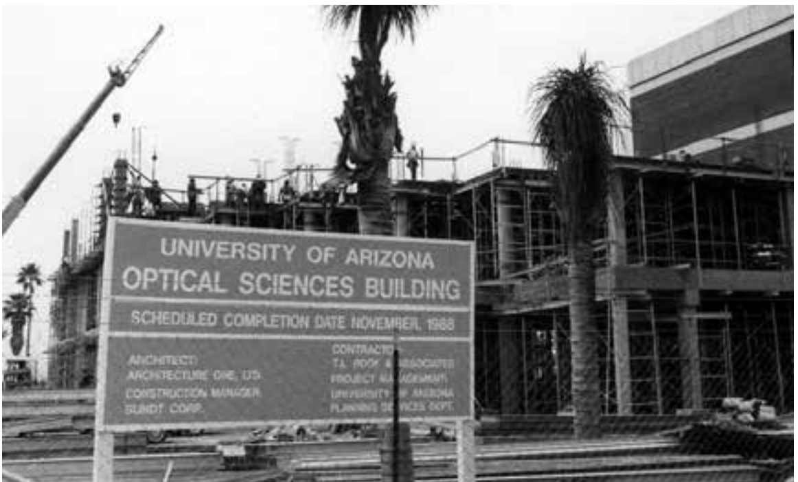
Construction of east wing, 1987.
