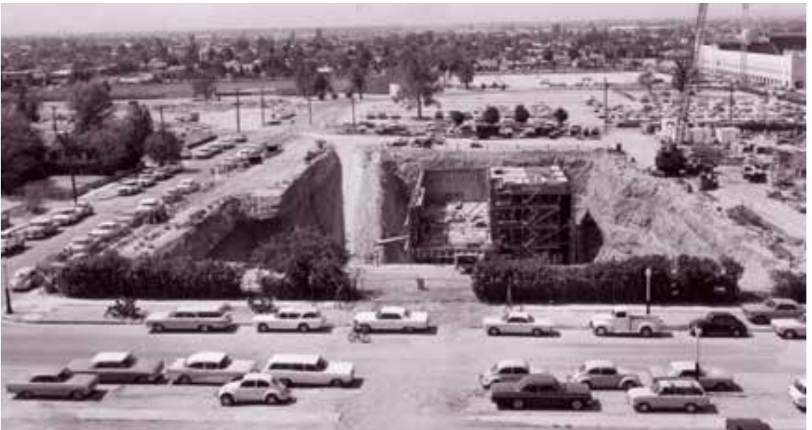
Initial construction on Optical Sciences Center building, 1968.
