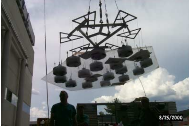
Figure 13. The completed facesheet, hanging from its whiffle tree.
